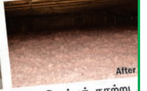
Blowing insulation
