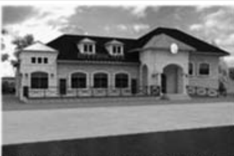
BUILD YOU DREAM RESTAURANT WITH THE BUILDING PERMIT $699,900
