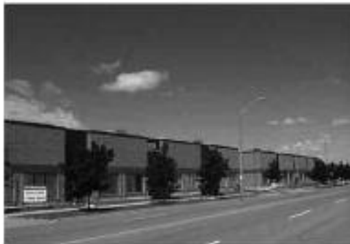
Warehouse ,industrial unit 8200 sq feet for sale asking 1050000
