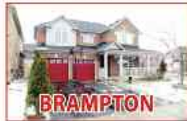
Airport Rd. & Brydon Blvd.
