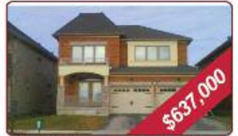
Ninth Line And Main Street Stouffville Bedrooms - 4, Washrooms - 3 Concept, 9' Ceiling, Hard Wood Floor Through The House
