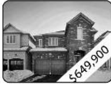
4 Bedrooms, 4 W Room Very Large Fully Fenced Backyard Close To School
