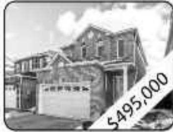
$495,000 3+1 Bedrooms, 4 W Room Professionally Finished Basement Seperate Entrance
