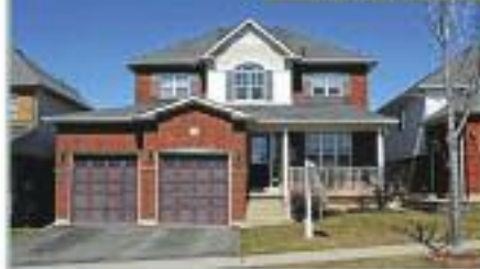
Oshawa - Wilson/Clearsky 3 Bedrooms, 3 Washrooms
