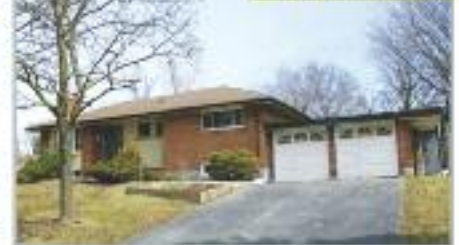
Toronto - Pharmacy/Sheppard 3 + 2 Bedrooms, 3 Washrooms Basement Finished
