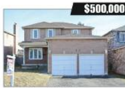
Ajax - Church / Delaney 3 Bedrooms, 3 Washrooms
