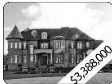
5 Bedrooms, 6 W Room Huge Rec Room In Fin W/O Bsmt W/ Above Grade Windows
