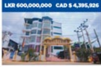
LKR 600,000,000 CAD $ 4,395,926 Luxurious Business complex For Sale in Kiramakottu Junction Point Pedro Land Size - 61 Perch • Total Sqft - 50,771
